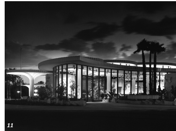
11. Valley National Bank, 44th Street and Camelback Road Photo courtesy: DWL Architects
