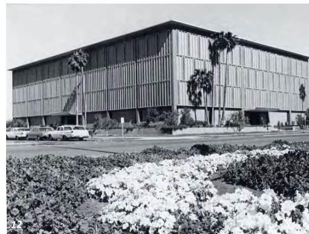
11,12. ASU Hiram Bradford Farmer Education Building by Reginald G. Sydnor with Edward L. Varney Associates, AIA - Tempe, 1960 Photo courtesy: University Archives Photographs, ASU
