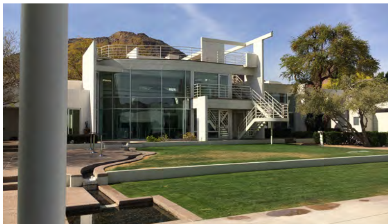
1. (previous page) Reginald G. Sydnor Photo: Duke Photography 2. (previous page) Cummings Exterior. Photo: Douglas B. Sydnor, FAIA 3. (above) Cummings Home from Backyard. Photo: Douglas B. Sydnor, FAIA
