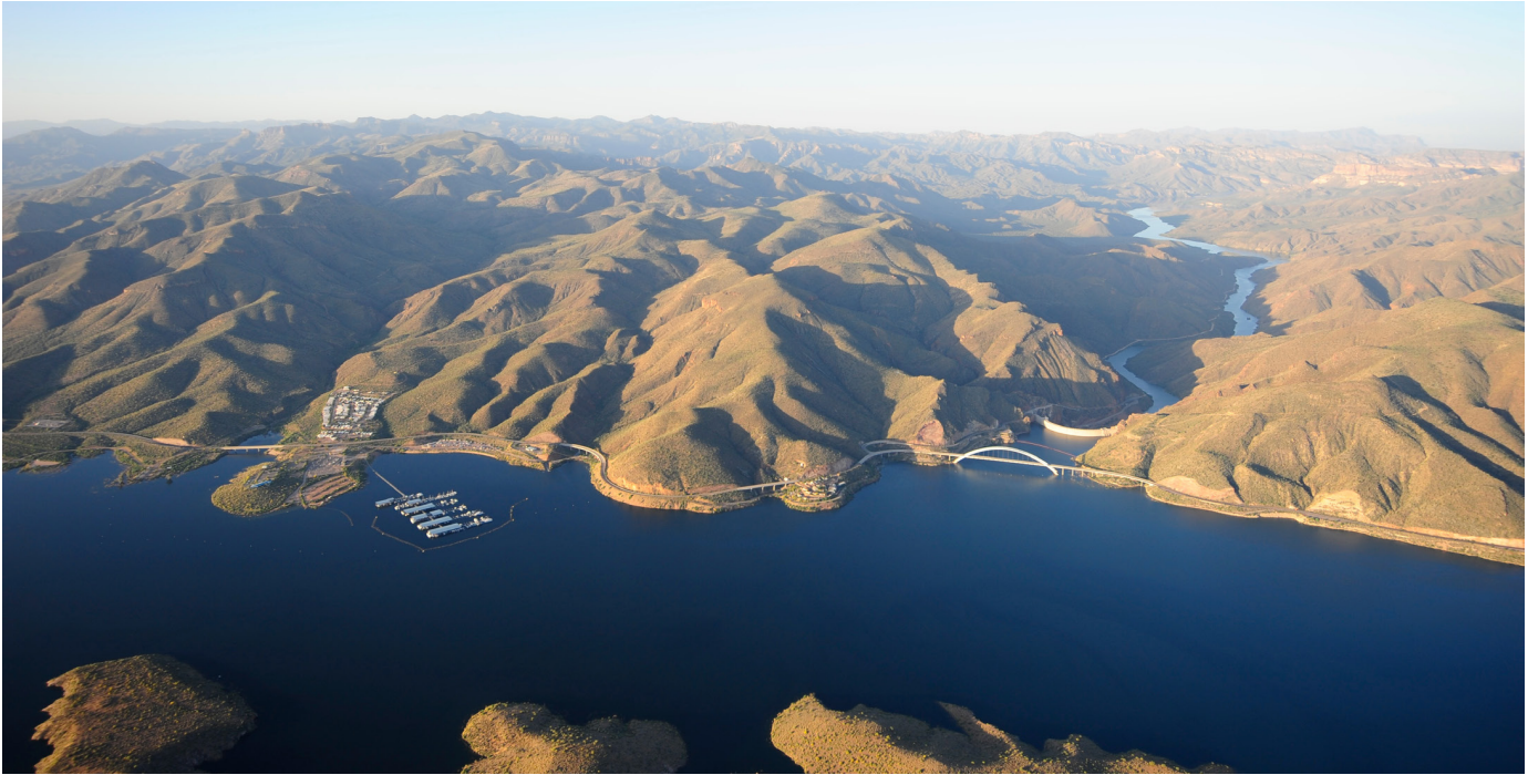
Built between 1905 and 1911, the Theodore Roosevelt Dam controls the once erratic flow of the Salt River and harnesses water for irrigation; it is the largest reservoir in the storage system for water and electricity provider, Salt River Project (SRP). Photo Courtesy of SRP.
