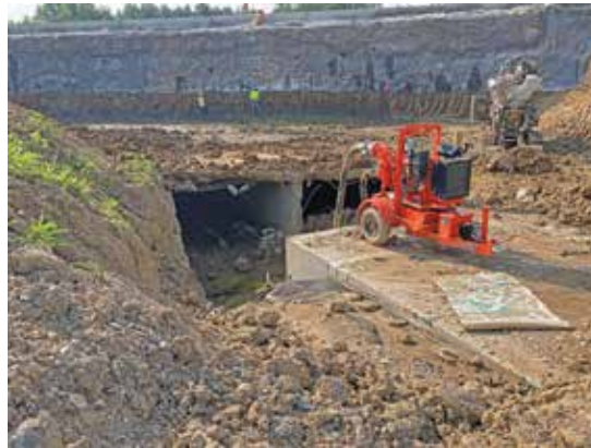
MOVING OUT Workers remove the original two-barrel box culvert under SR 67.
