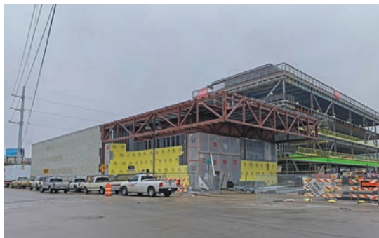
STRONG REMEMBRANCE The super-structure cantilevers over the entrance to Greenwood Rising.
